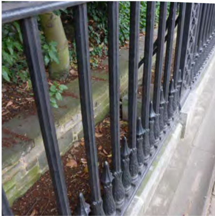
Left (York Terrace West): A third of the railings have been replaced to the east of the site. The repaired railings sit on a low parapet wall that matches the small section of replaced railings on the corner of York Terrace East.
