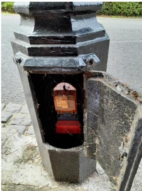
Figure 3-1 - Existing Lighting Column
