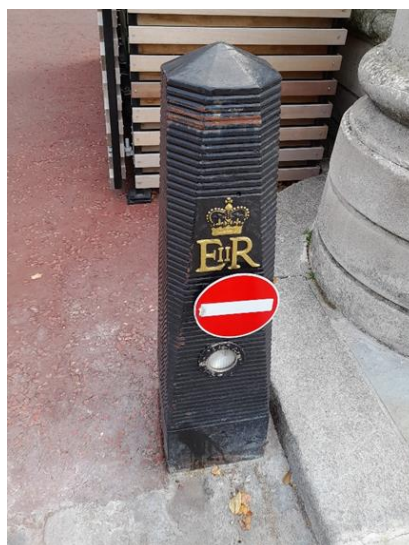
Figure 4-3 - Existing bollard with Queen Elizabeth cypher, complete with halogen spotlight
