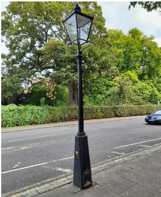
Figure 1-2 - Heritage style lighting column
