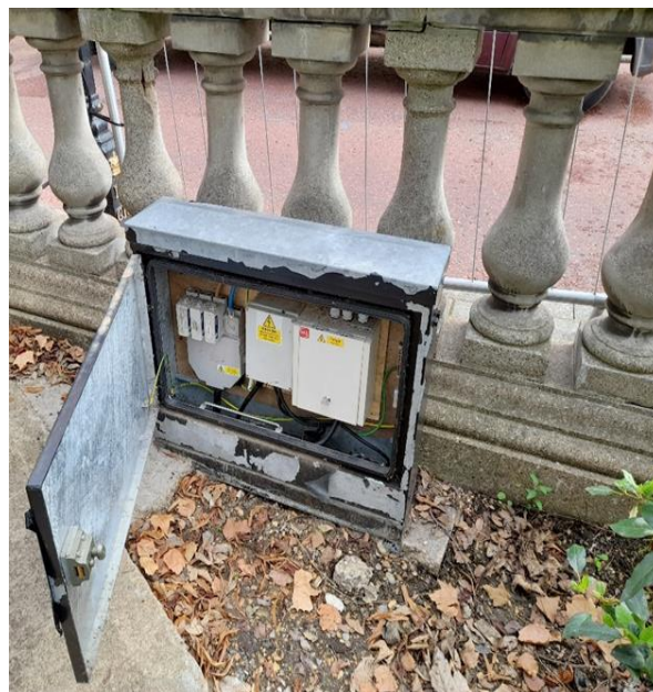
Figure 3-4 - Existing supply point at Chester Terrace
