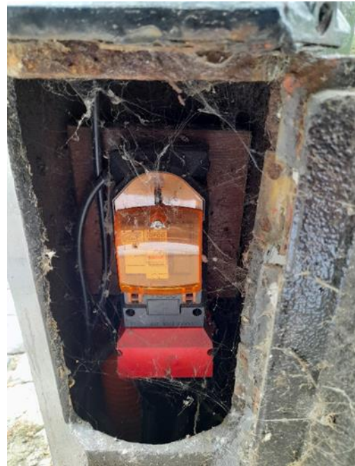
Figure 3-2 - Existing Column Cut-out
