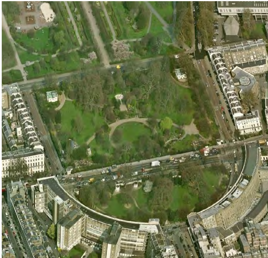
Fig. 6 Bird’s-eye View of Park Crescent and Park Square c.2012
