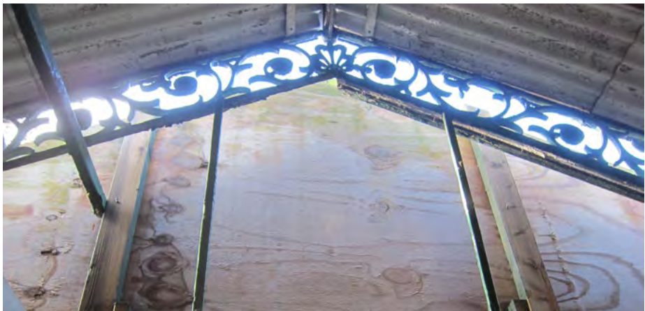
Right: Cast iron detailing visible on the west gable from inside the pavilion
