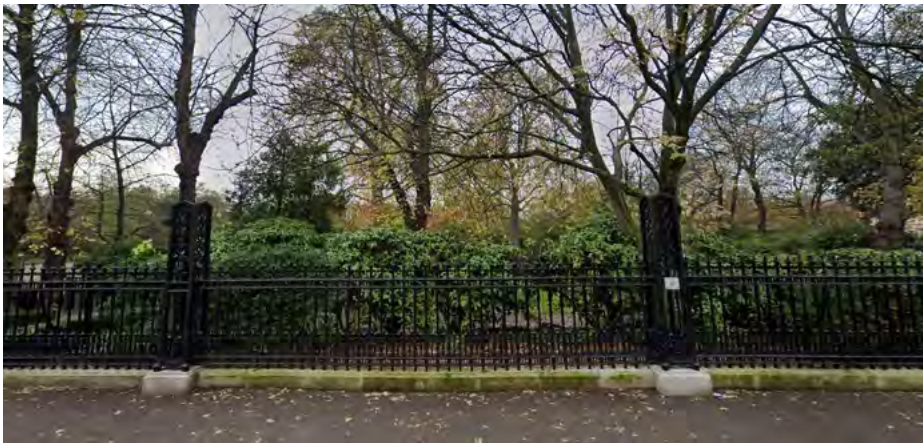
Right: Existing railings along Park Square East
