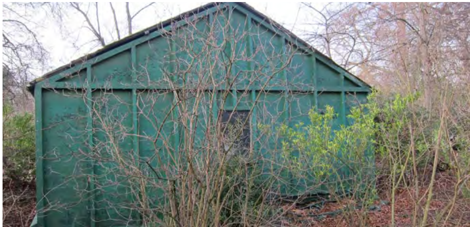
Right: The ironwork pavilion in Park Square has been boarded and is currently used as a storage shed
