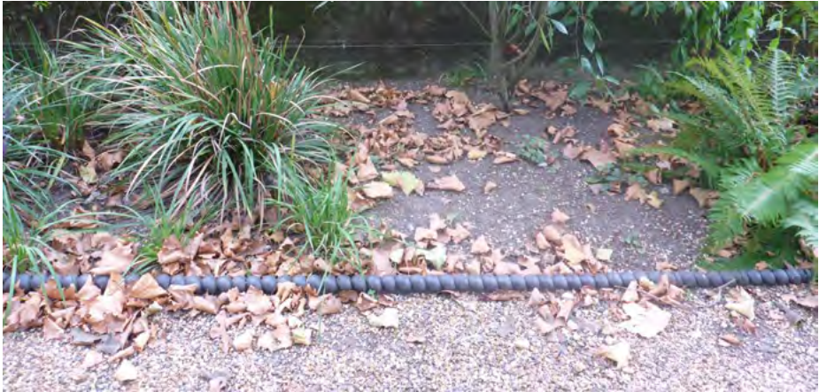
Rope edging is a common feature in most of the terraces and, when installed correctly, provides an attractive and practical barrier for vegetation and gravel.
