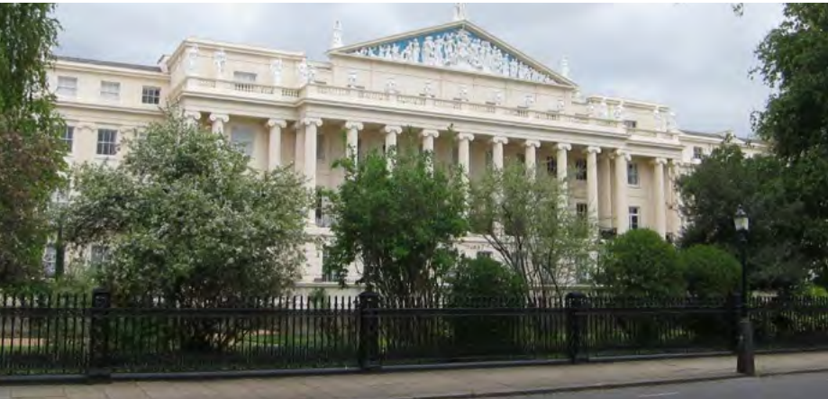
Existing view from the opposite site of the Outer Circle. Tall shrub planting acts as a screen to the terrace beyond.
