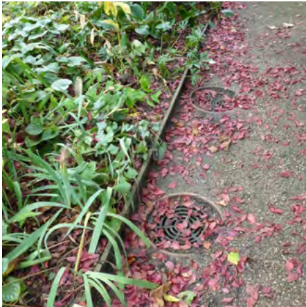
Far Left: Tight curves are hard to achieve using rope edging and therefore it is better suited to straight sections
