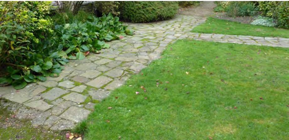
Left: Piecemeal changes to the original gravel paths have resulted in an incongruous mixture of surfaces. Sections of crazy paving are an incongruous addition to the garden that are at odds with the grandeur of the building.
