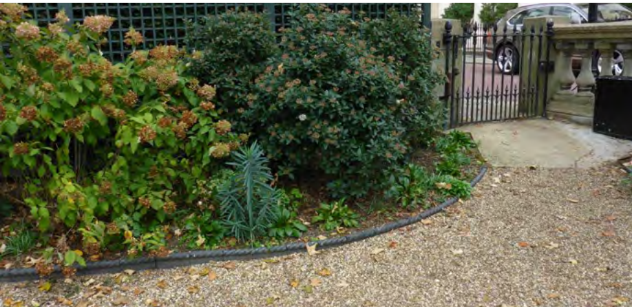
Rope edging is a common feature in most of the terraces and when installed correctly, provides an attractive and practical barrier for vegetation and gravel.
